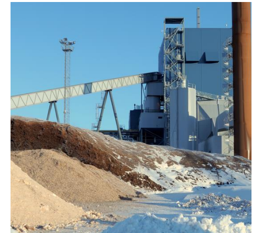
Typical multifuel CHP plant in Finland. Photo: VTT
