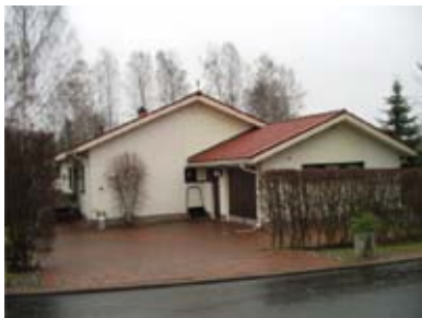
Figure 2.2 New building completed approx. 2–3 years after receiving a building permit
