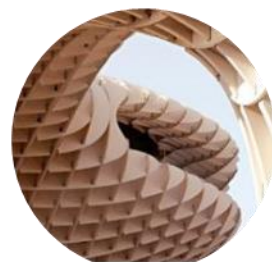
Building and living
